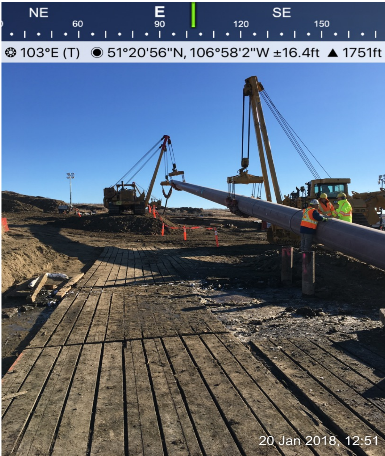
TAIL END OF THE BORE BEING PULLED
