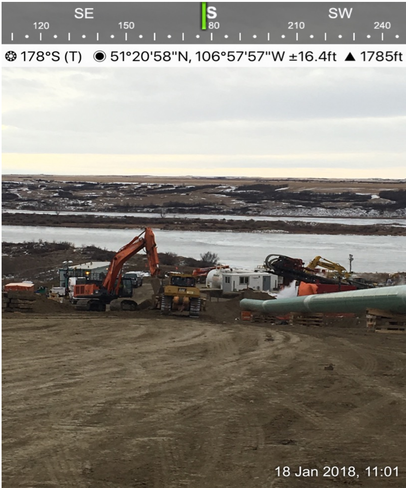
CREW MOVING SOIL PILE OUT OF THE WAY FOR DRAG SECTION
